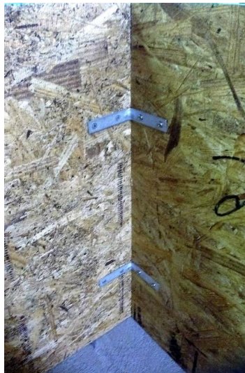
Figure 11: Exterior of Walls Joined using Angle Brackets, Bolts, and Wing Nuts
