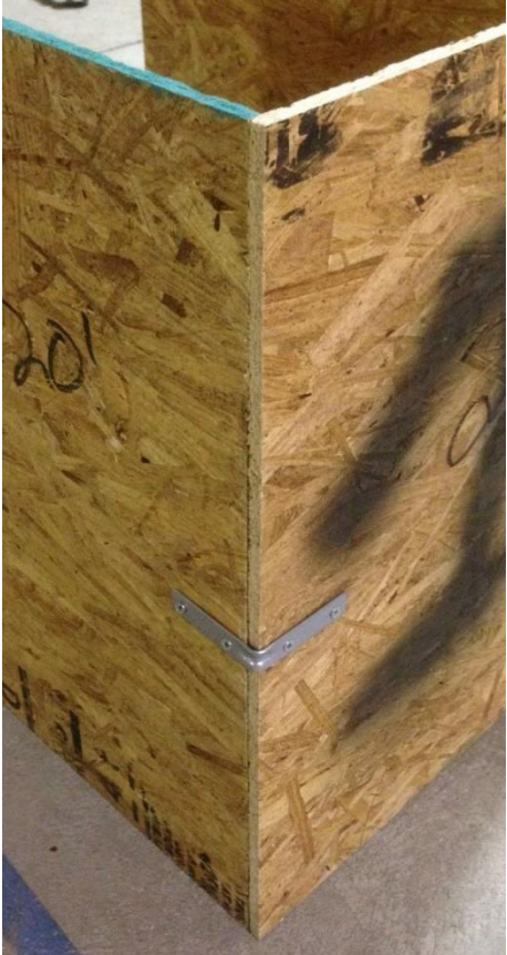
Figure 4: Exterior Angle Bracket of Protrusion
