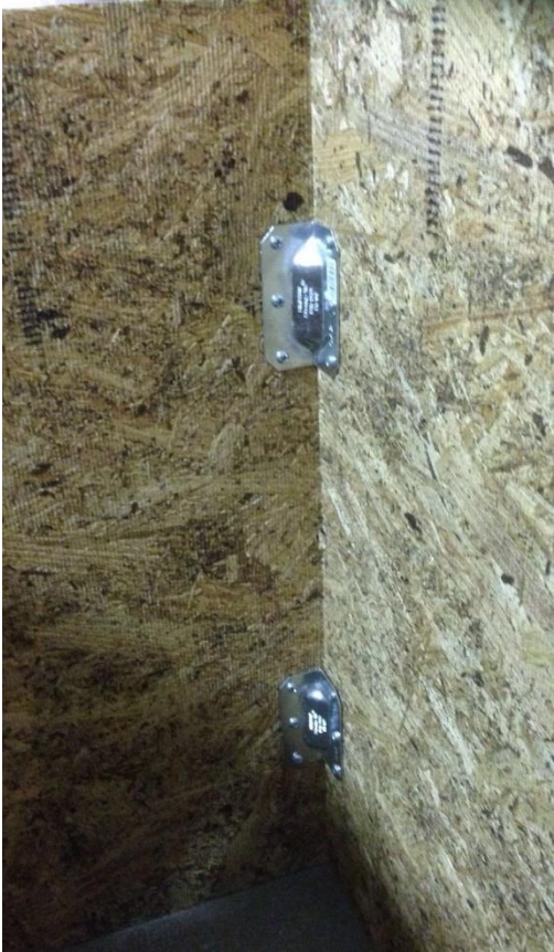
Figure 3: Interior Angle Brackets of Protrusion
