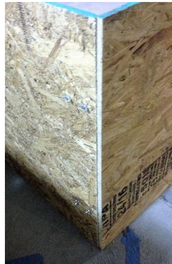
Figure 12: Interior of Walls Joined using Angle Brackets, Bolts, and Wing Nuts
