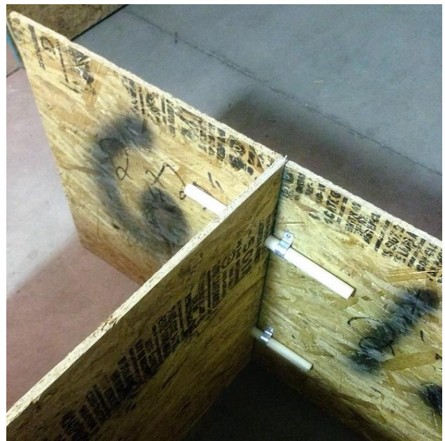
Figure 7: Spot Dowel Connectors
