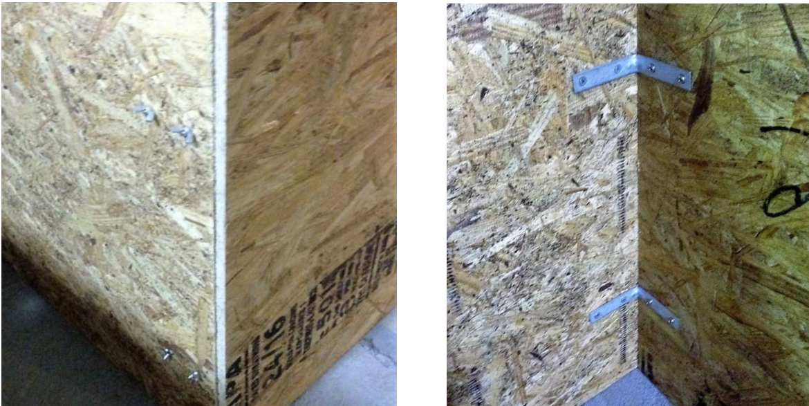
Figure 2. 90 degree brackets for parking walls (Courtesy: Dorothy)
