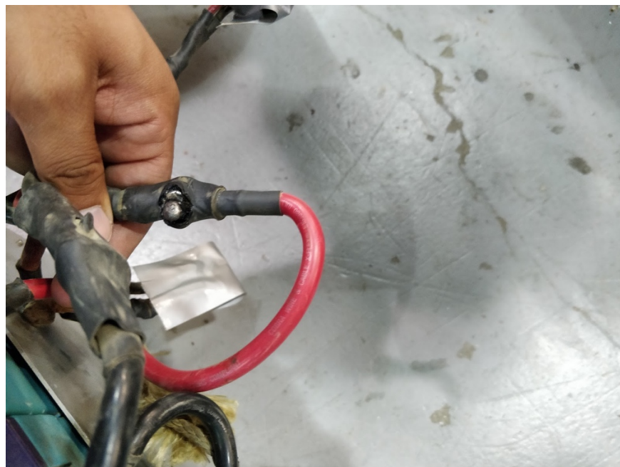
Figure 1 Damaged Battery Cable
