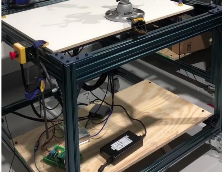
Figure 5: Electrical Setup Under Table
